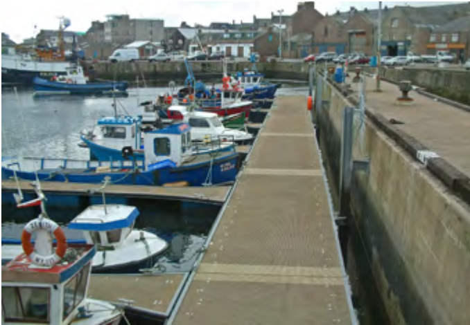
Peterhead Harbour, Port Henry Basin Pontoons
