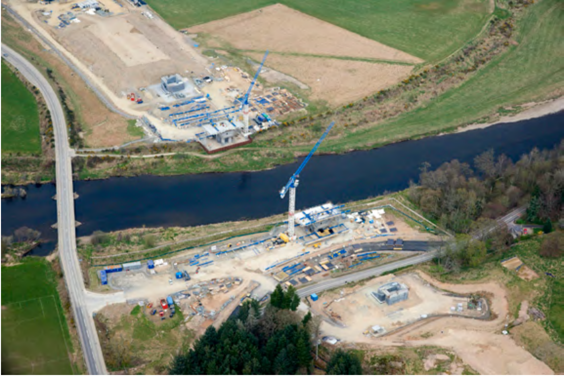
There are 78 bridges across the length of the project
