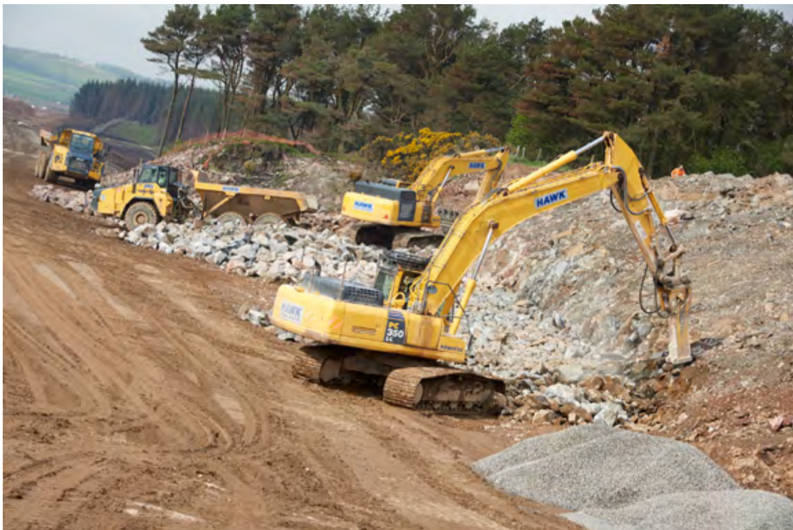
During maximum earthworks, 230 dump trucks, 150 excavators and 60 dozers were used
