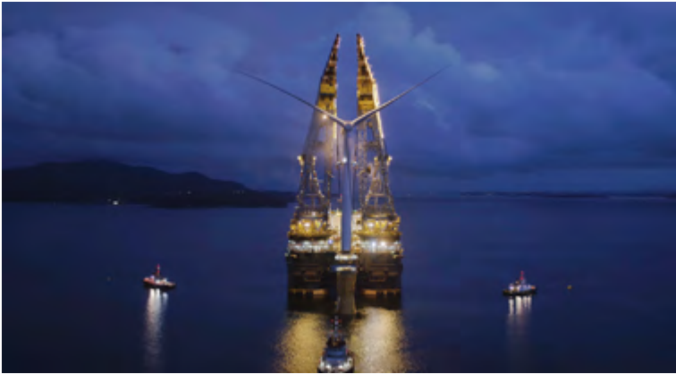
Statoil Hywind mating of turbine to spar foundation prior to arrival in Peterhead Image courtesy of Statoil
