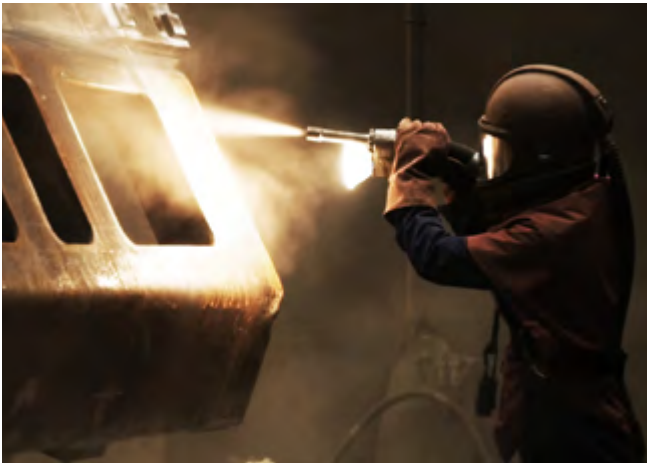
Blast cleaning steel Image courtesy of Davidsons Blast Services Ltd., Peterhead
