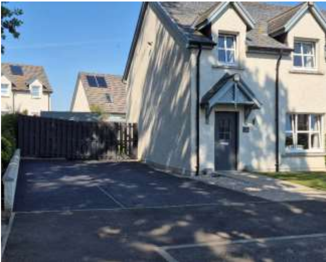
Front of House and Driveway
